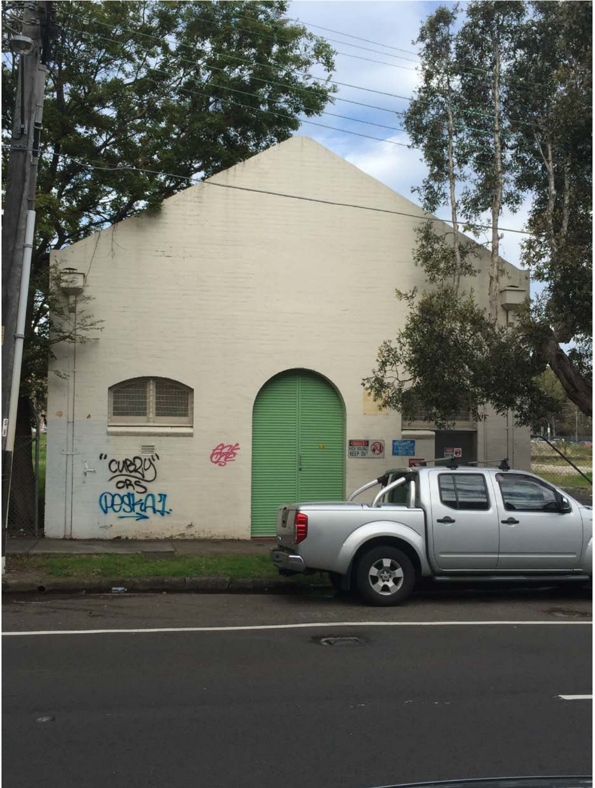
Figure 10: Ausgrid Heritage listed Sub Station – Young Street
