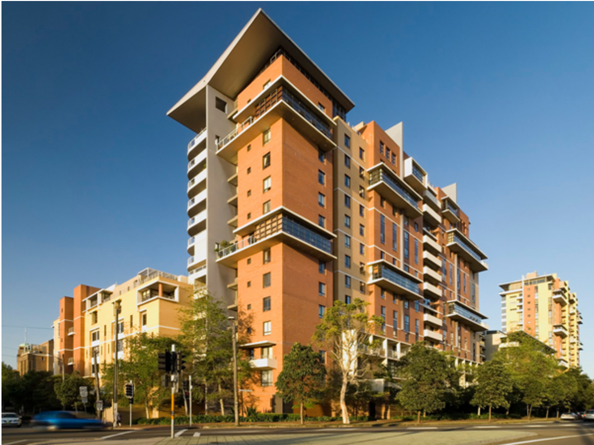
Figure 14: Moore Park Gardens Development, corner of Phillip and Bourke Streets
