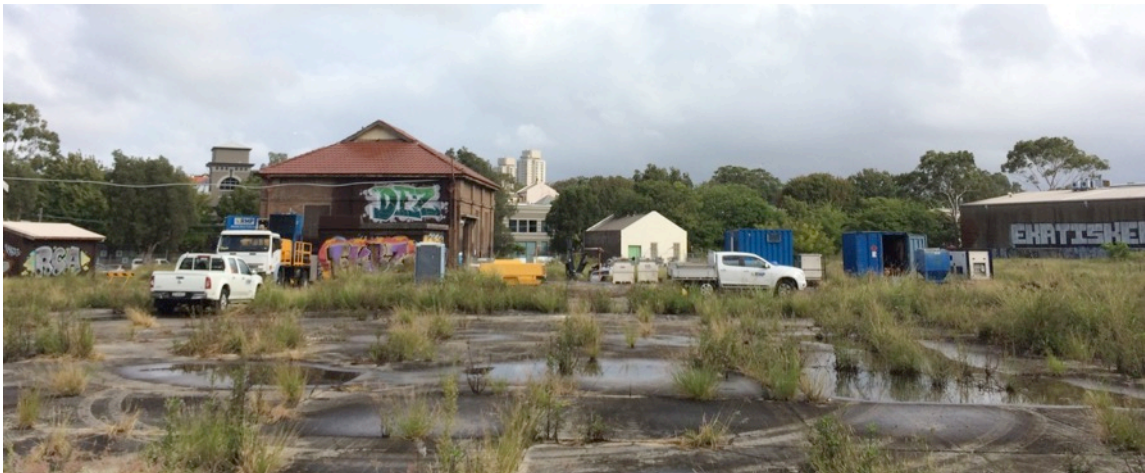
Figure 2.33: View to rear elevation of Electricity Substation No.18 from Bourke Street.
