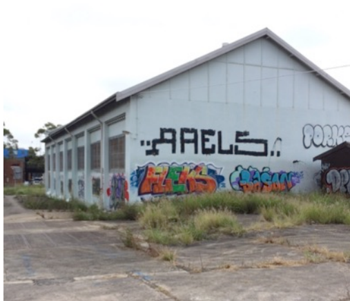
Figure 2.9: Rear (northern elevation), Pumping Station
