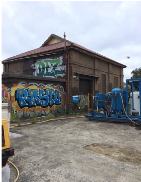
Figure 2.18: Exterior, Valve House
