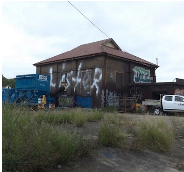
Figure 2.19: Exterior, Valve House
