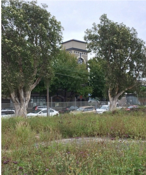
Figure 2.37: View to 222 Young Street from land adjacent to Pump & Valve Houses
