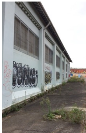
Figure 2.10: Eastern elevation, Pumping Station
