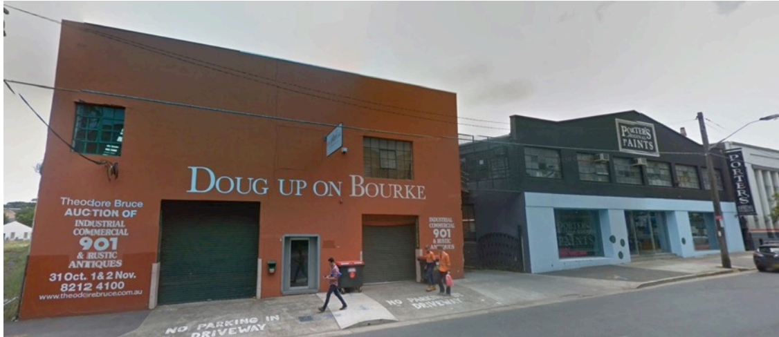
Figure 2.41: 895-901 Bourke Street, Waterloo, 2015 Source: City West Housing website
