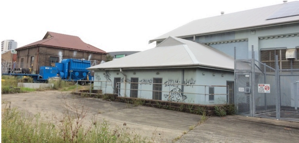
Figure 2.17: View towards Pump House and Valve House from southwest.
