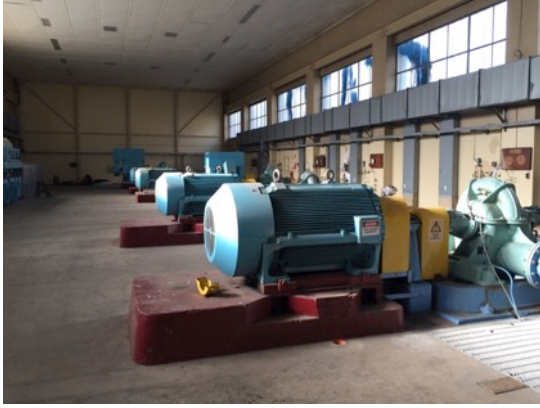
Figure 2.12: Interior, Pumping Station, 2015. Source: Dahua via City of Sydney
