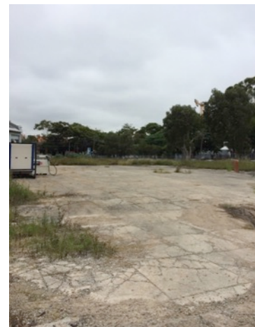
Figure 2.29: View across site, showing evidence of the location of former buildings
