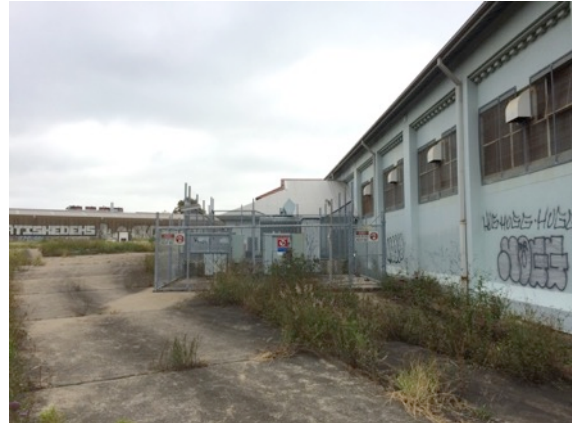
Figure 2.6: West elevation, looking towards north, showing substation and 1960 extension, Pumping Station
