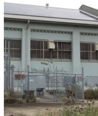
Figure 2.11: Detail, west elevation, showing dentils and steel-framed windows, Pumping Station
