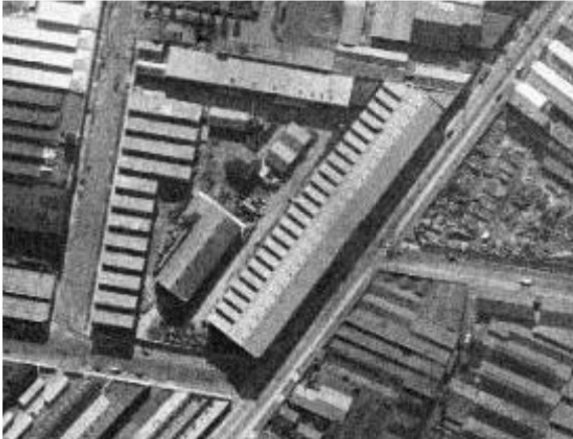
Figure 2.24: Central workshops, surrounding the Pump and Valve Houses in 1943. Source: NSW LPI Six Maps
