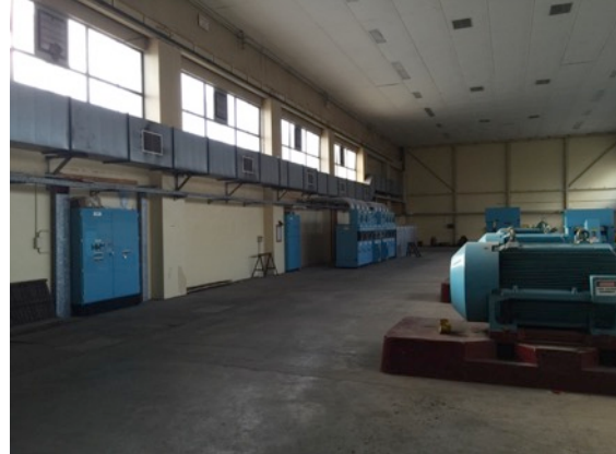
Figure 2.13: Interior, Pumping Station, 2015. Source: Dahua via City of Sydney
