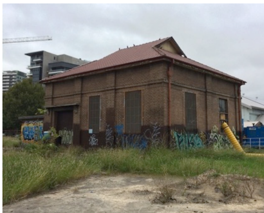
Figure 2.20: Exterior, Valve House
