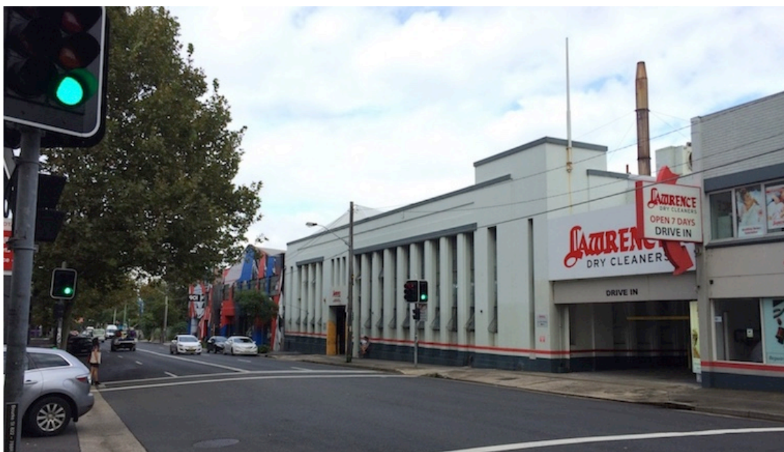
Figure 2.43: part of 887-893 Bourke Street
