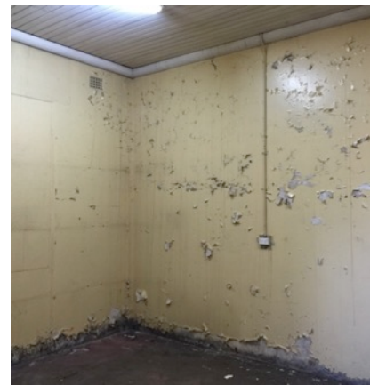
Figure 2.16: Interior, 1960 extension, Pumping Station, 2015. Source: Dahua via City of Sydney
