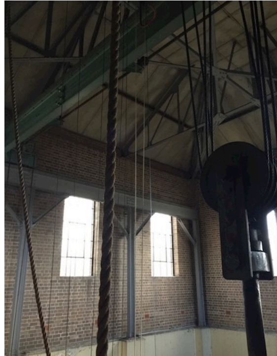
Figure 2.23: Interior, Valve House, 2015. Source: Dahua via City of Sydney
