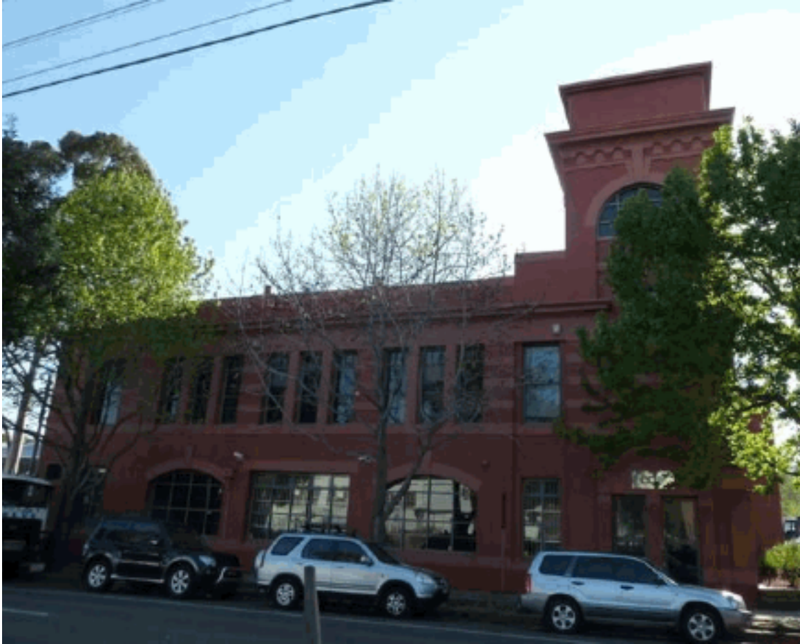
Figure 2.34: 222 Young Street, Waterloo, c2012 Source: State Heritage Inventory
