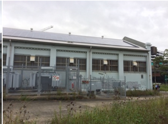
Figure 2.8: Substation, western elevation, Pumping Station
