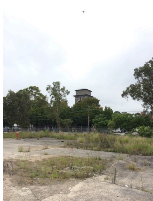
Figure 2.38: View to 222 Young Street from land adjacent to Pump & Valve Houses
