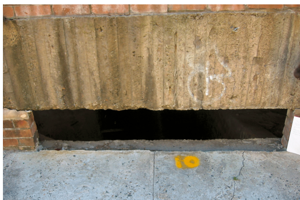
Photo 4: Inlet point for overland flow into stormwater channel downstream of South Dowling St and Lenthall St low point Photo 5: View through inlet in Photo 4, looking downstream at stormwater channel.
