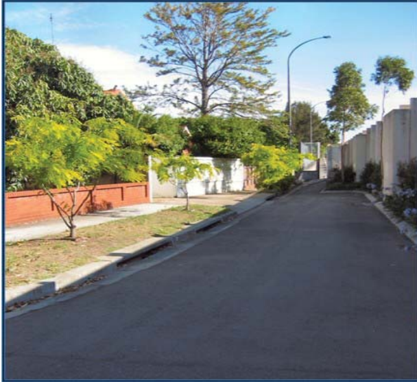
Photo 1: Inlet Pits near South Dowling and Myrtle Streets West Kensington.
