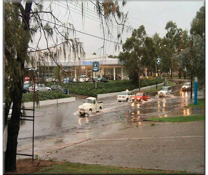
Photo 2: Minor Flooding (0.3 m depth) observed in Joynton Avenue trapped low point following a small storm in February 2001.
