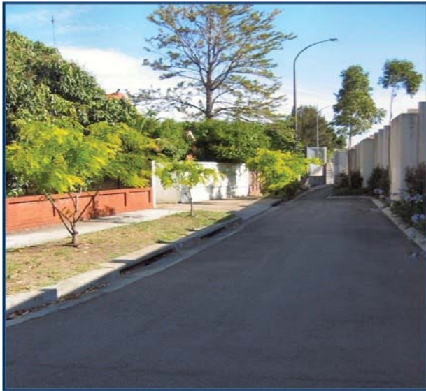
Photo B1: Inlet Pits near South Dowling and Myrtle Streets West Kensington.
