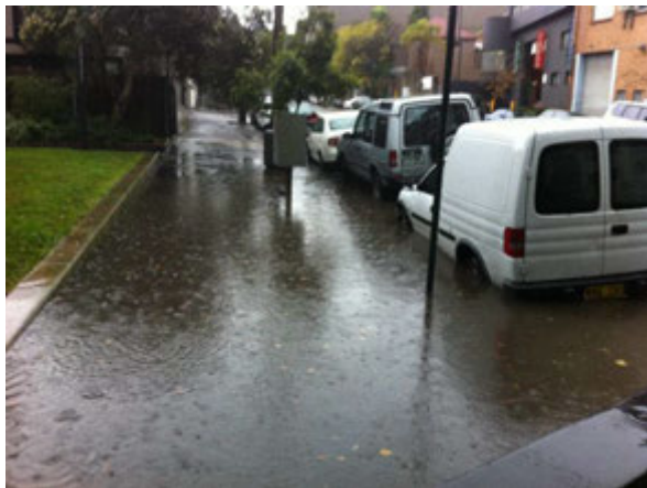
Photo 1: Flooding on Sparkes Street.
