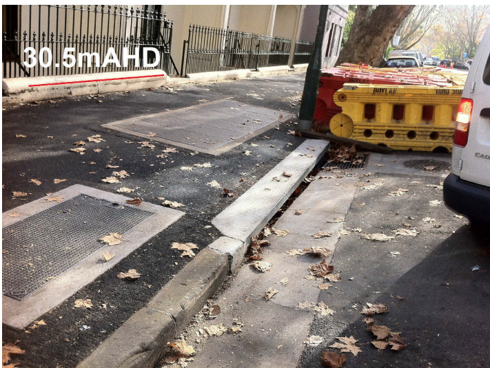
Approximate elevation of flooding on Victoria St during June 2007 storm.
