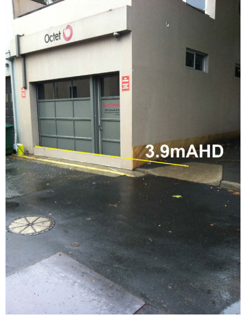
Flood barrier installed at Bossley Terrace, with approximate elevation of barrier height.
