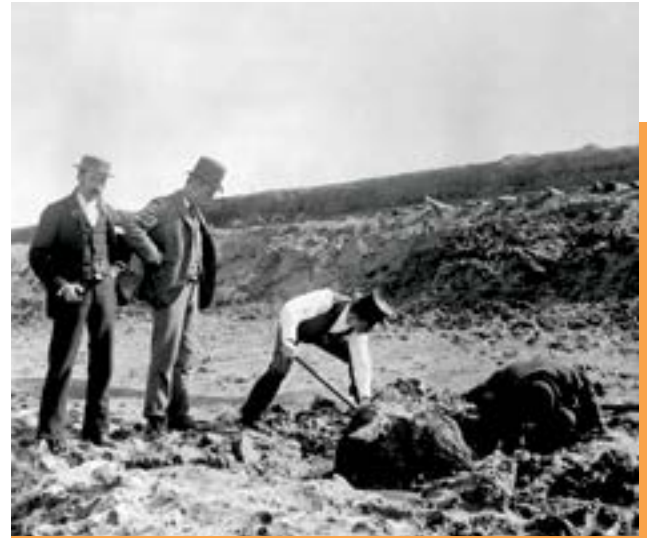
Excavation at Sheas Creek in 1896 (photograph courtesy Australian Museum)
