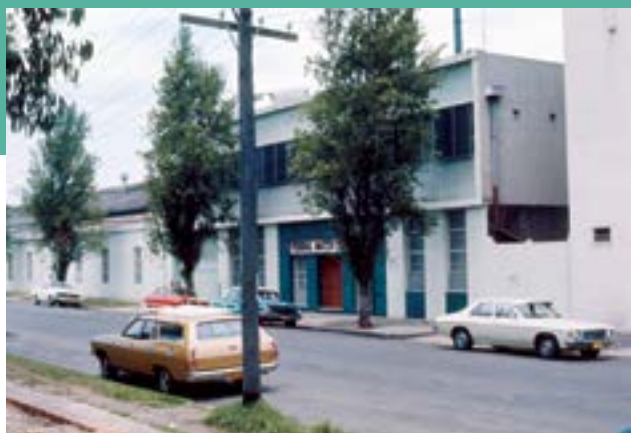
34 FEDERAL MATCH FACTORY, 7-11 PARK ROAD, ALEXANDRIA
