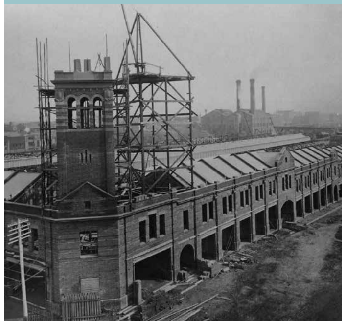
Fruit Market under construction, 1911 (Photograph: City of Sydney Archives)
